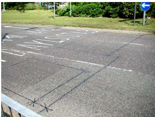
Figure 3. Example of a mounting of an inductive loop in the road
