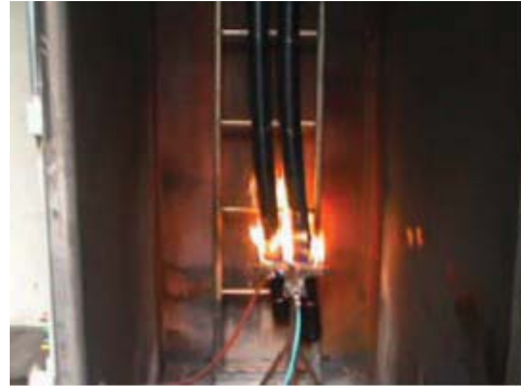
Figure 7. Fire test of high voltage cables.
