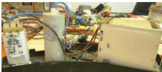
Fig. 1. Sample public lighting component in Dakar.
