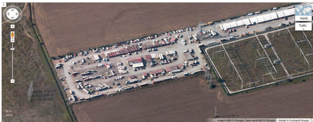
Fig. 2. The market place adjacent to the substation and converging power lines (Google Maps)
