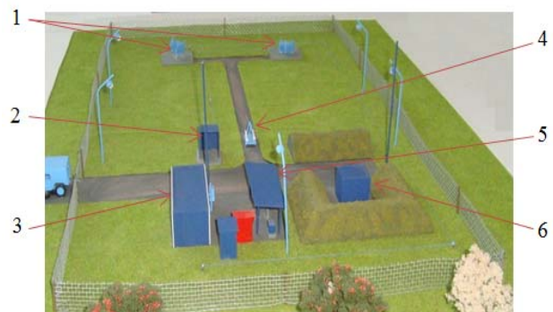
Fig. 1. Structure of local anti-hail unit: 1- suppression missiles launch ramps; 2- command point for missiles launch; 3- box housing; 4- missiles transport trolley; 5- technical point; 6- missiles depot.
