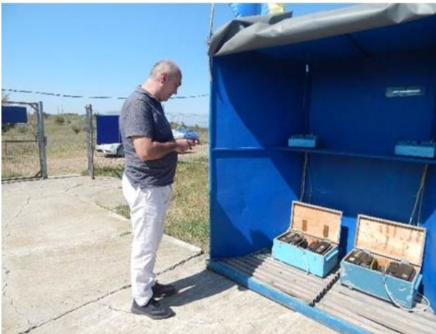
Fig. 4. Batteries of a missile launch site
