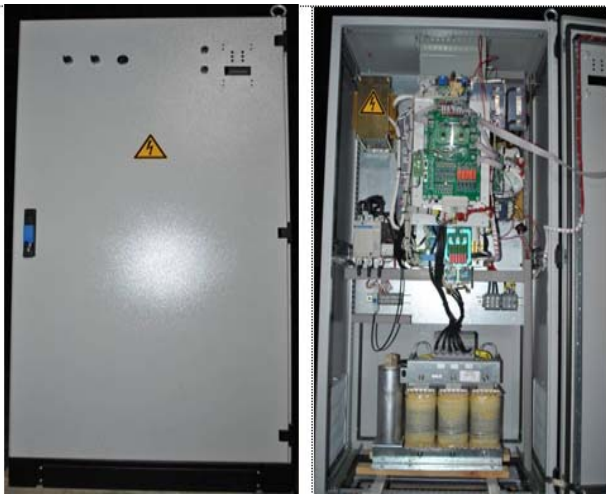
Fig. 14. The achieved construction of the power unit with variable voltage and frequency.
