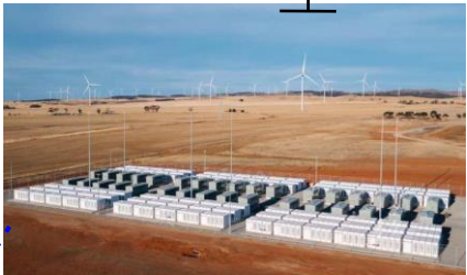
Energy Storage System
