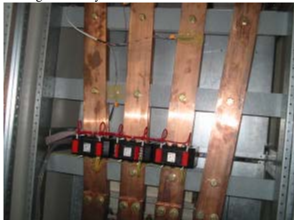
Figure 12. The emplacement of sensors
