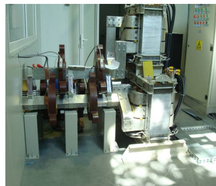
Fig. 8. Source output busbar system
