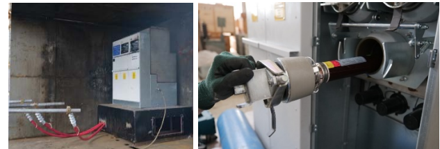
Fig. 12. Distribution switchgear in experimental circuit for pressure testing. Fuse placement on a side phase.
