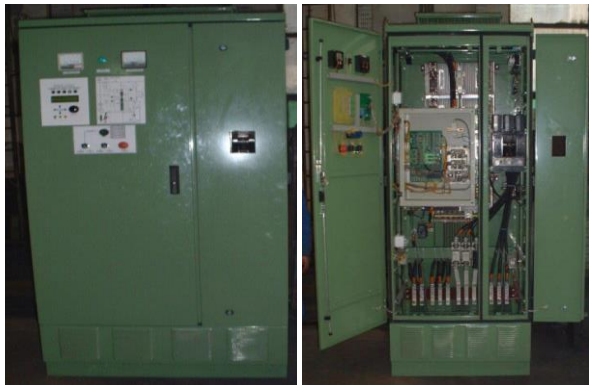
Fig. 3. The equipment cabinet Eex-MS 500V/500A-01
