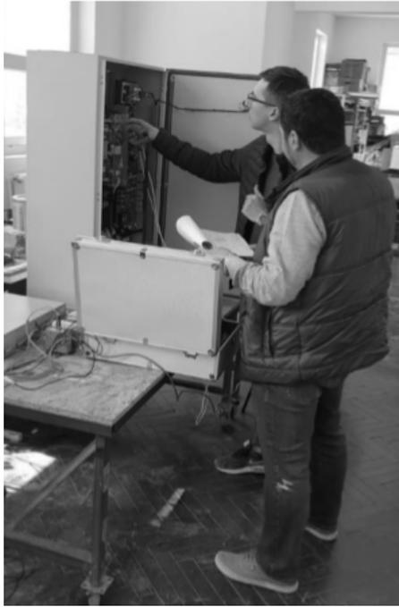
Fig. 4. Current and voltage transducers mounting.
